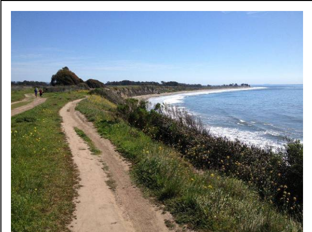
The blufftop trail section of the Coastal Trail is the second most heavily used trail section on Ellwood Mesa. The trail is located very near the bluff edge and is below grade resulting in the creation of gullies and potholes as well as erosion from surface water runoff over the bluff.
