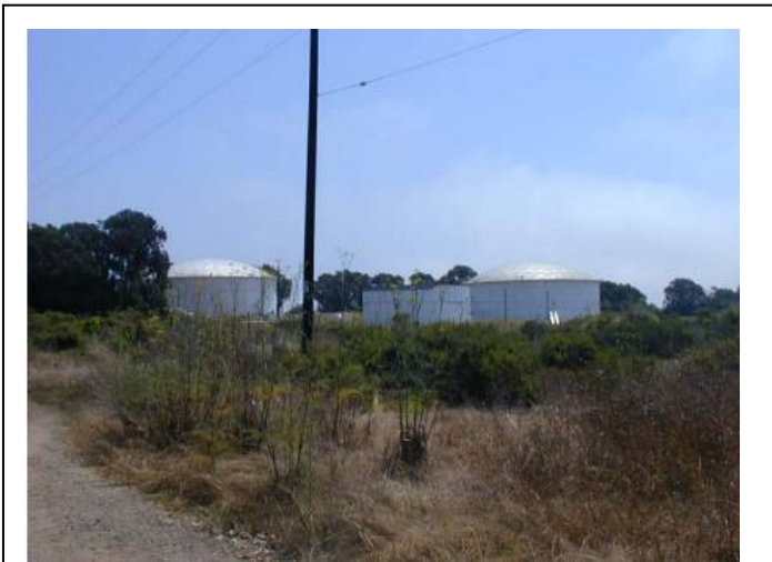
The Ellwood Marine Terminal, operated by Venoco, is located adjacent to the west of the Project area, occupies 17.5 acres, and receives and stores crude oil.
