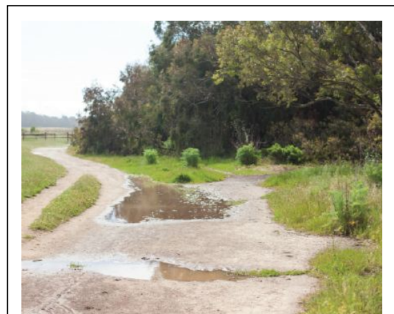
"Braiding effect" on the existing Ellwood Mesa trail network due to user bypass of poorly drained surfaces.
