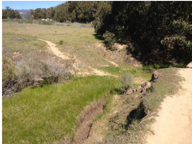
Topography in the vicinity of the Devereux Creek as well as the gullies within the Ellwood Mesa Open Space Plan Area is characterized by grades exceeding ten percent. These steep grades exceed safety thresholds and can make the trail inaccessible for some users.
