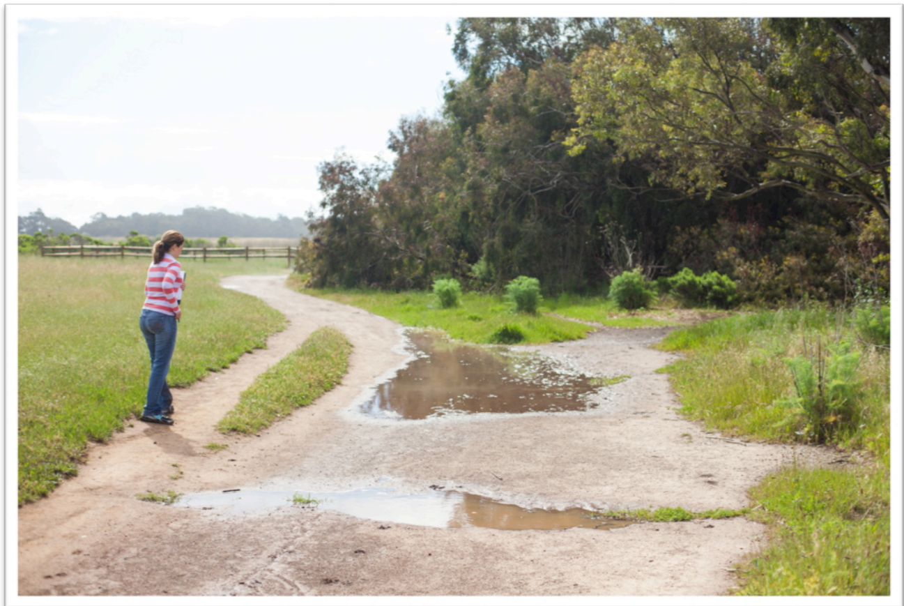
Photo above shows the bluff-top trail proposed for improvements. The trail is below grade and as a result water pools along it. Braided trails have cropped up as a result, widening the trail and impacting the vegetation.
