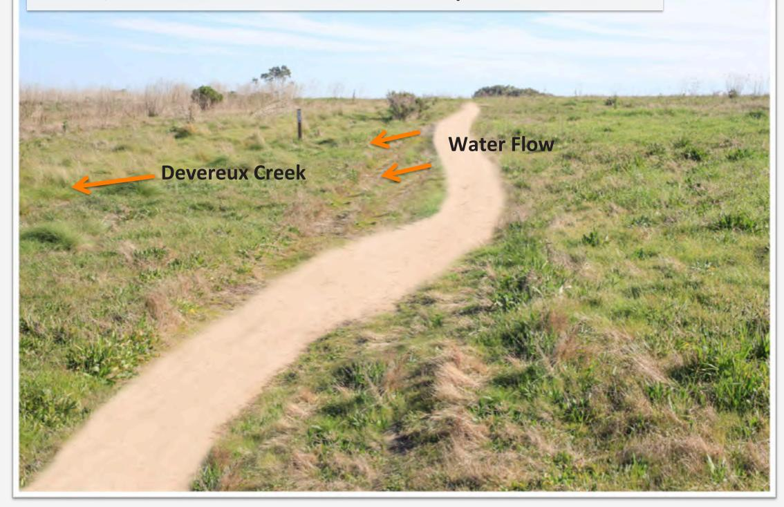
Trail is entrenched (below surrounding area) about 8-10" and water can only flow down it. Small adjustments like those shown in previous slide can minimize erosion and create a pleasing flow.
