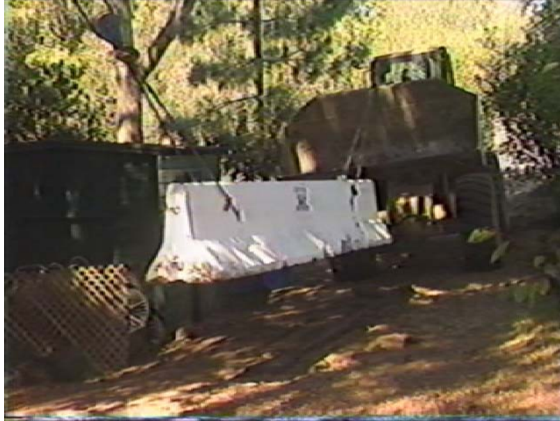
Figure 3 – Placement of K-Rail after the Painted Cave Fire in 1990
