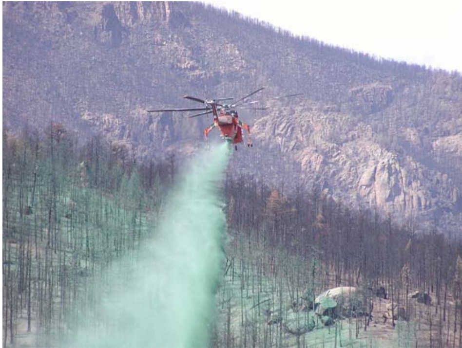
Figure 4 – Aerial Hydromulching (USFS, Colorado 2002)
