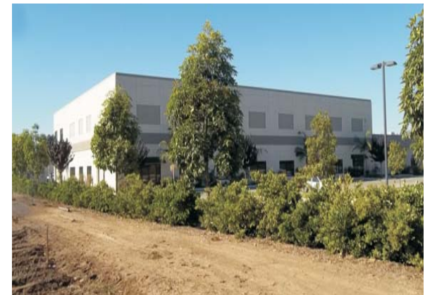
Photograph 12: View of the western adjoining commercial property, facing southwest.
