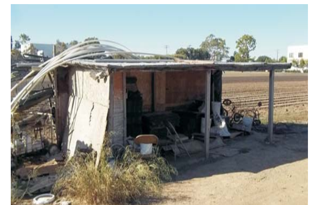
Photograph 6: View of the makeshift structure and materials storage area on the central portion of the subject property, facing southeast.
