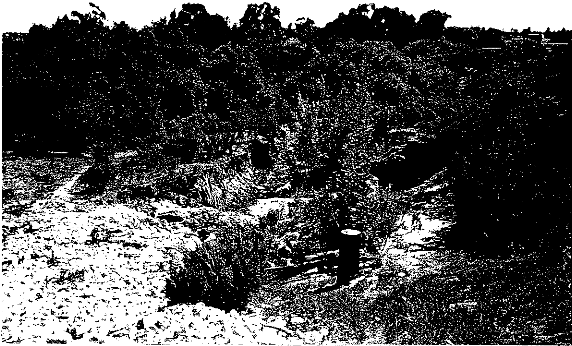
Photo 27. Outlet for overflow pipe at base of dam, looking south from east end of dam. Erosion of this area occurred during record rainfall season of 1997/98, resulting in significant sediment inflows to the overflow pond. Photo taken 7 April 1999.
