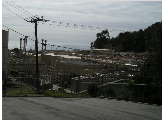
Venoco Ellwood Onshore Oil and Gas Processing Facility
