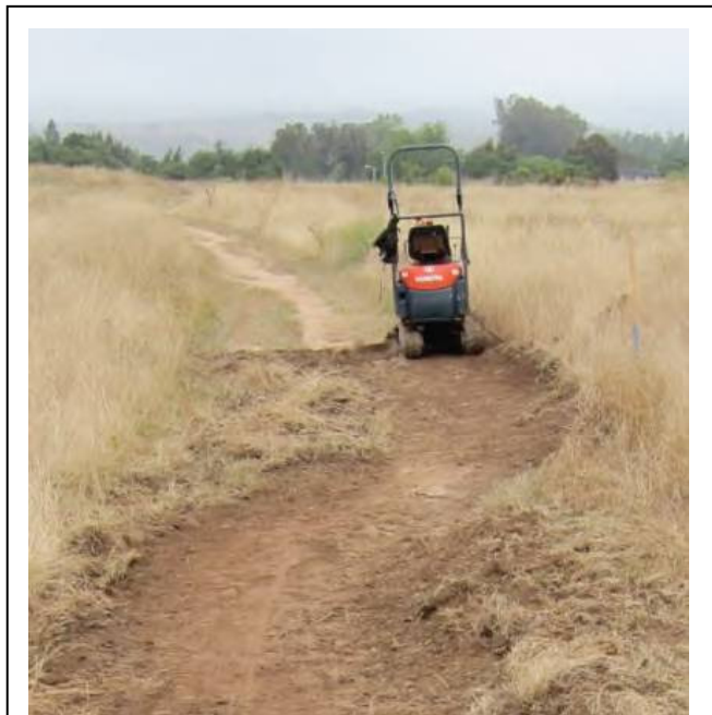
Limited heavy construction equipment would be required for recontouring of the trail surface (such as the equipment shown above, used for minimal trail disturbance at Lake Los Carneros). (Photograph courtesy of Ray Ford)
