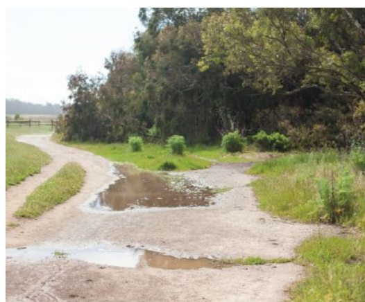
"Braiding effect" on the existing Ellwood Mesa trail network due to user bypass of poorly drained surfaces.
