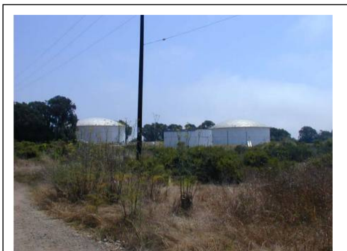
The Ellwood Marine Terminal, operated by Venoco, is located adjacent to the west of the Project area, occupies 17.5 acres, and receives and stores crude oil.
