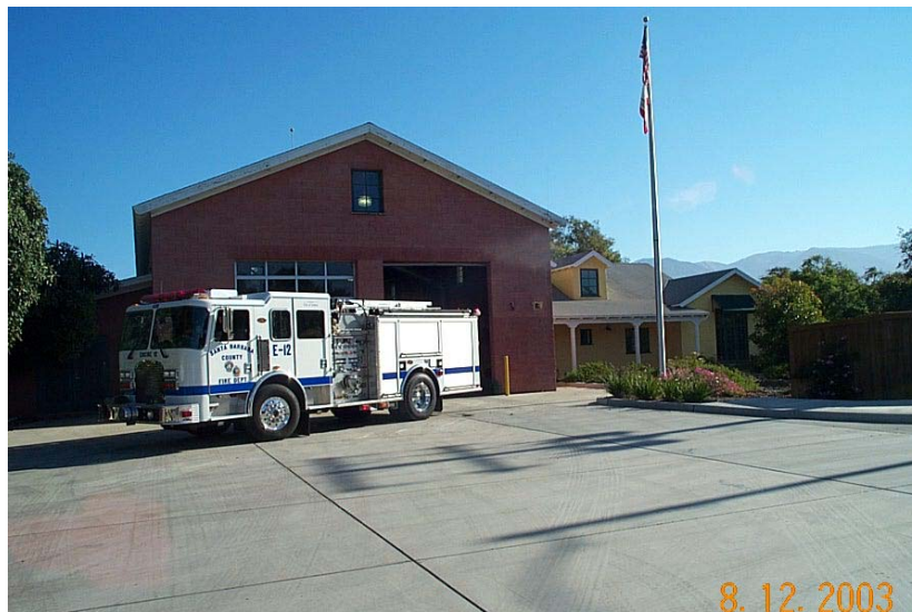
Photo courtesy of Santa Barbara County Fire Department
