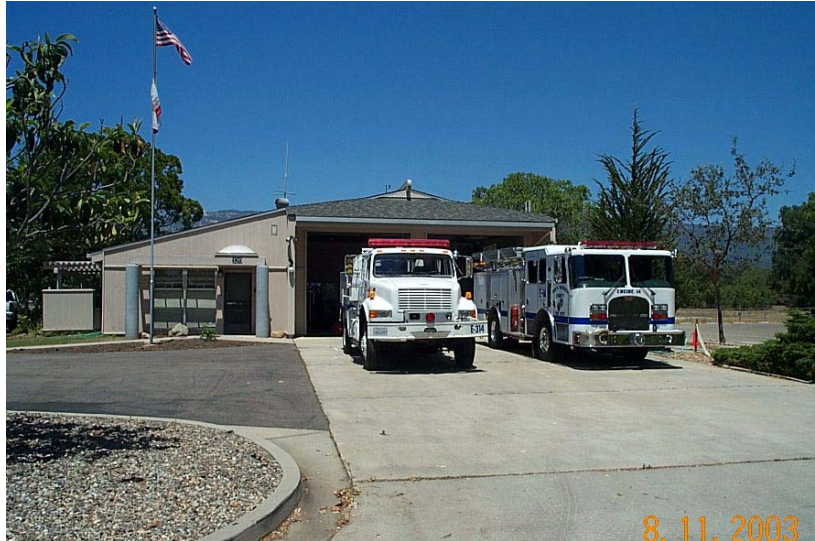
Photo courtesy of Santa Barbara County Fire Department
