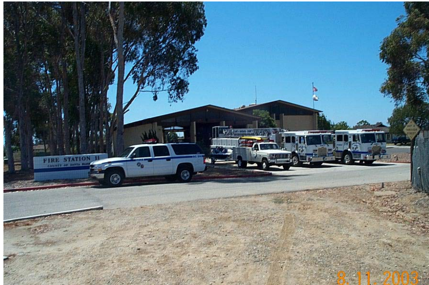
Photo courtesy of Santa Barbara County Fire Department
