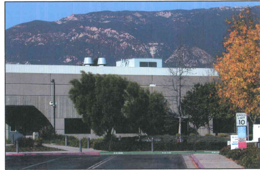
EXISTING FRONT OF BUILDING
