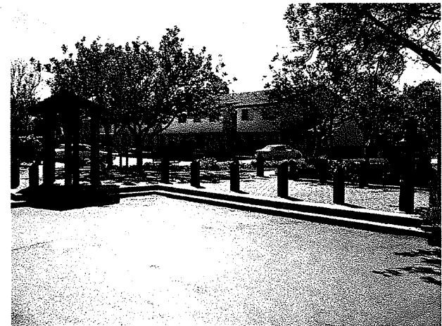
Grade difference at entry
