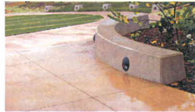
Colored concrete with score joints
