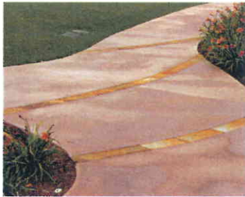
Colored concrete with stone banding
