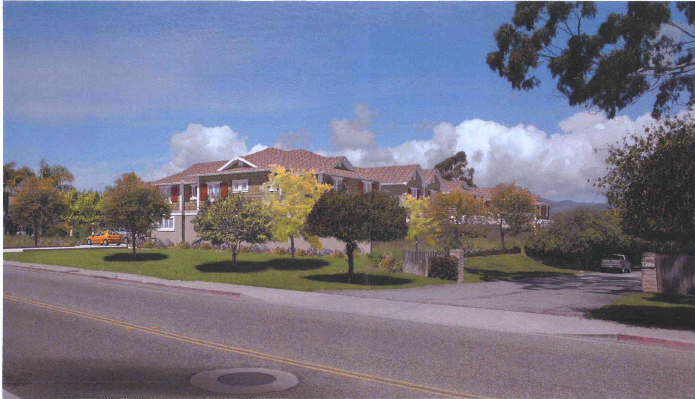
SOUTH EAST CORNER ACROSS CALLE REAL
