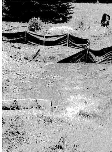
Figure 1: DDT contaminated stormwater breaching site BMPs and carrying pollutants through neighboring residences to Carpinteria State Beach.
