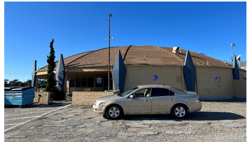
Photograph 4. View of the existing building, facing west.
