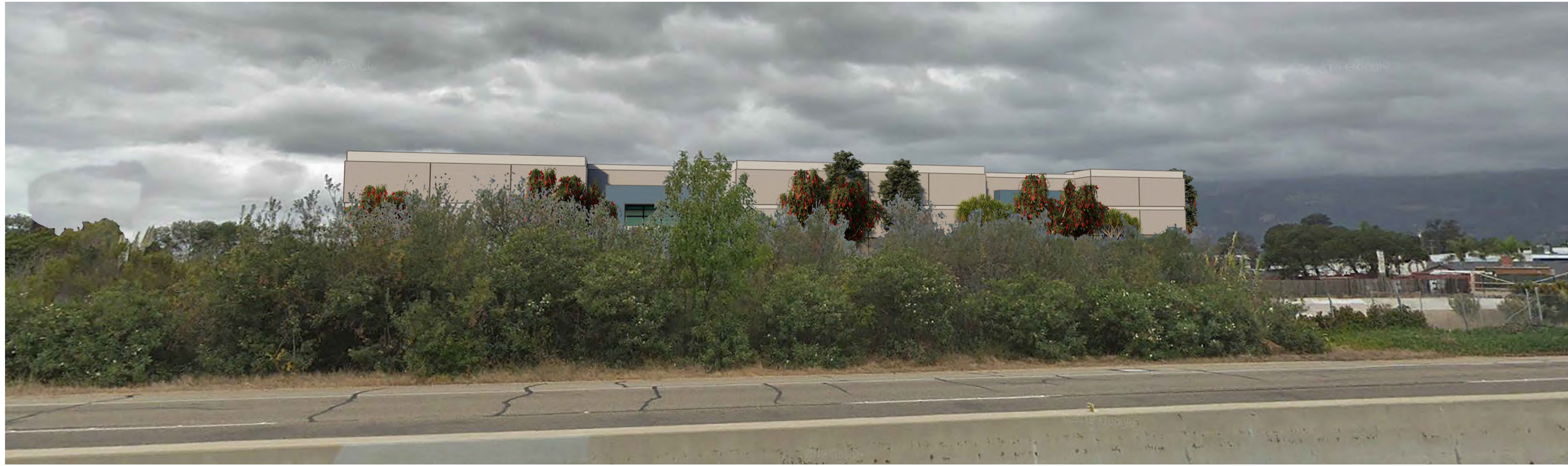
① VIEW FROM HIGHWAY 217
