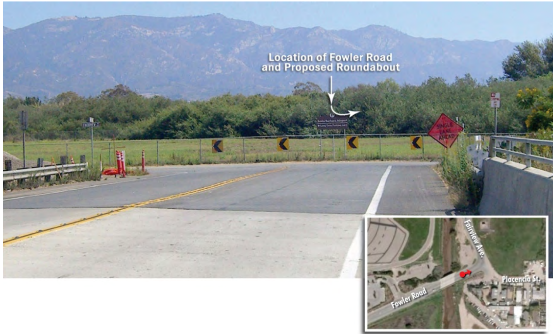
Existing view of proposed Fowler Road extension location as viewed by an eastbound traveler on Fowler Road
