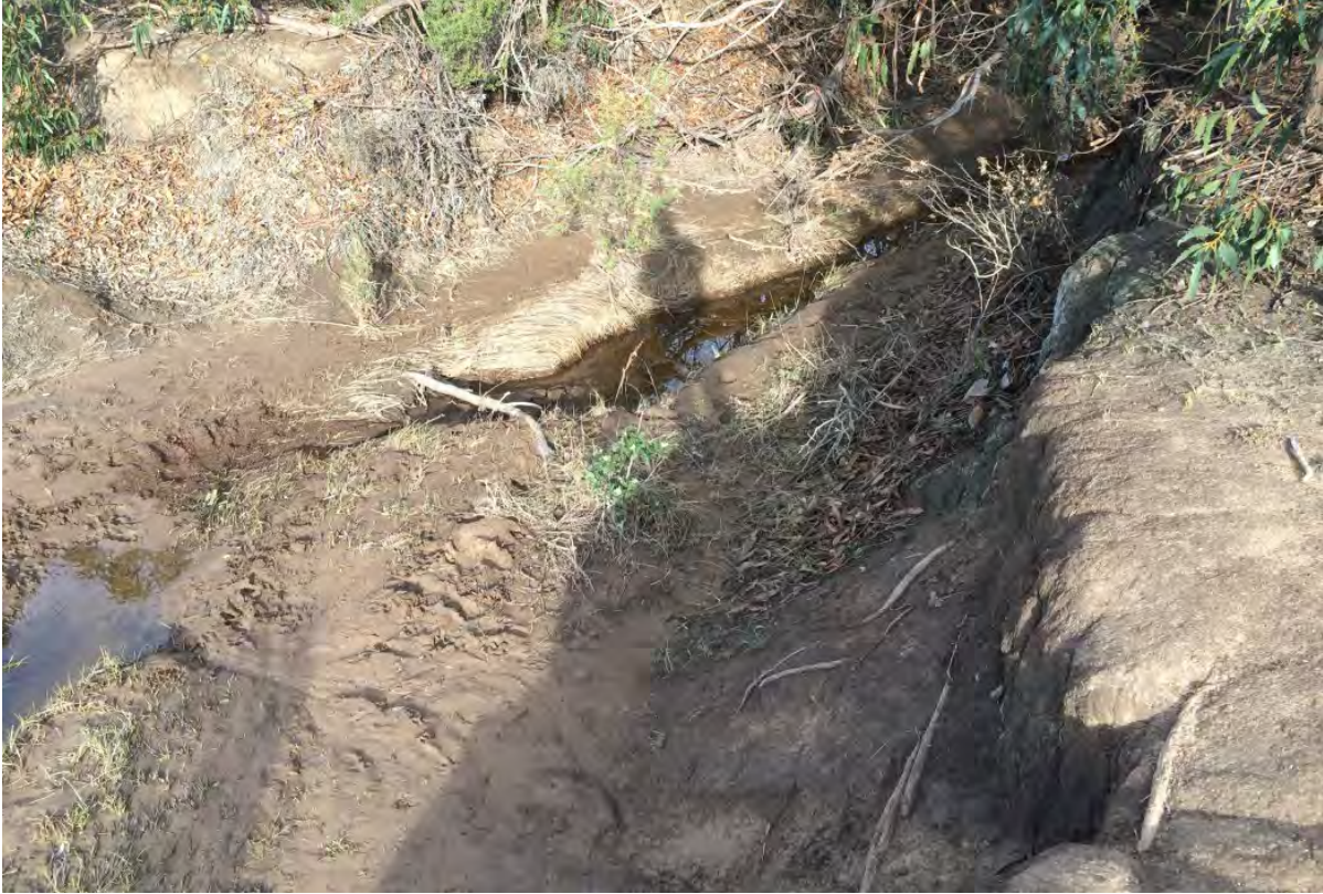
Photograph 3. View of tributary of Devereux Creek east of Kestrel Lane facing northwest (downstream). January 11, 2016
