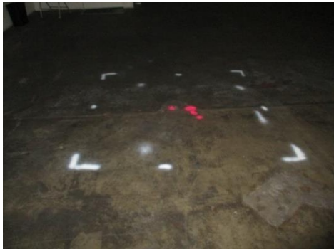
GPR investigation of pipes in the floor in the southeast corner of the west warehouse space.
