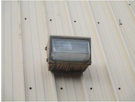
Mercury, sodium, or halogen light on exterior of building.
