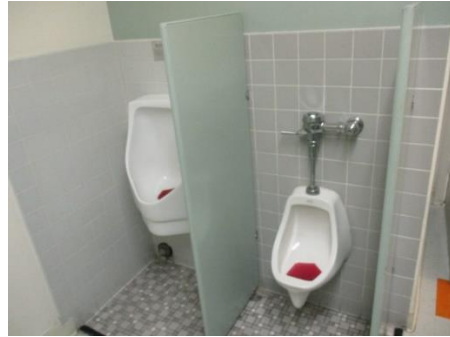
Lead-laden ceramic wall trim in the men's bathroom behind and next to urinals
