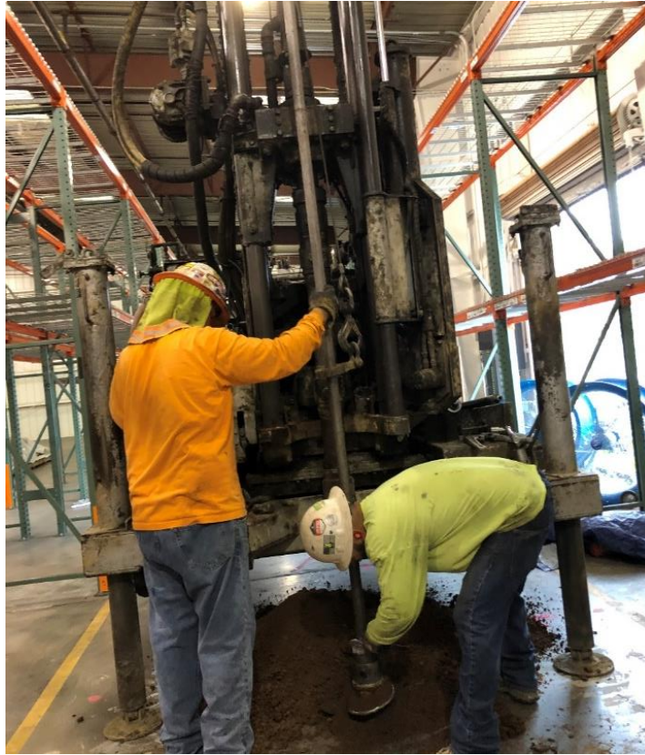
PHOTO 2.3.2-1: Boring Inside Existing Warehouse
