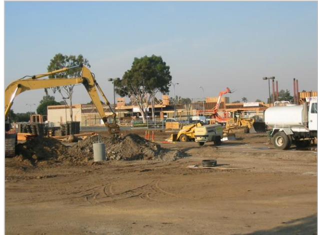
Heavy Equipment at a Construction Site
