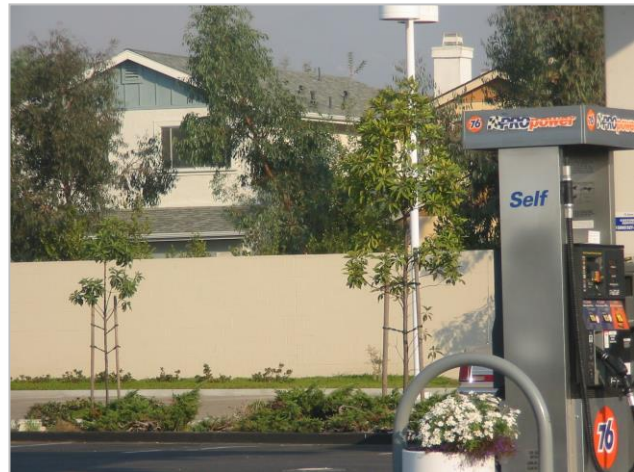
Sound Wall Separating Residential and Commercial Developments
