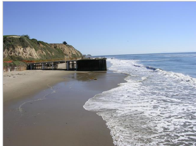
Piers Associated with Oil Production along the Shoreline Adjacent to the Sandpiper Golf Course
