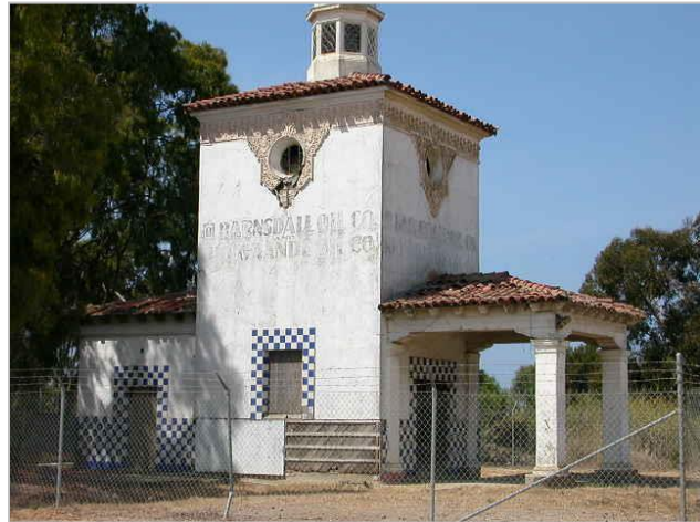
1929 Barnsdall-El Rio Grande Gas Station on Hollister Avenue
