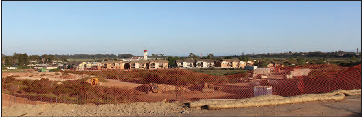
Current Conditions Without Simulated Road Construction
