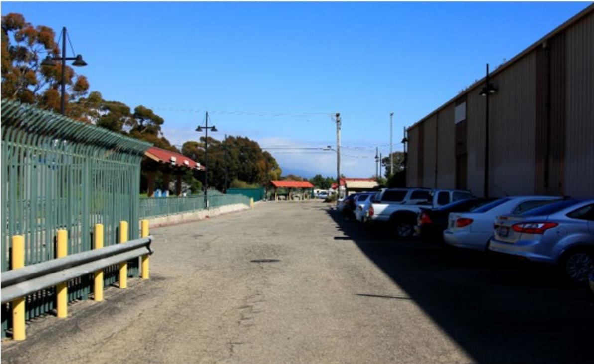
View of the north side of the existing building looking east along the railroad right-of-way
