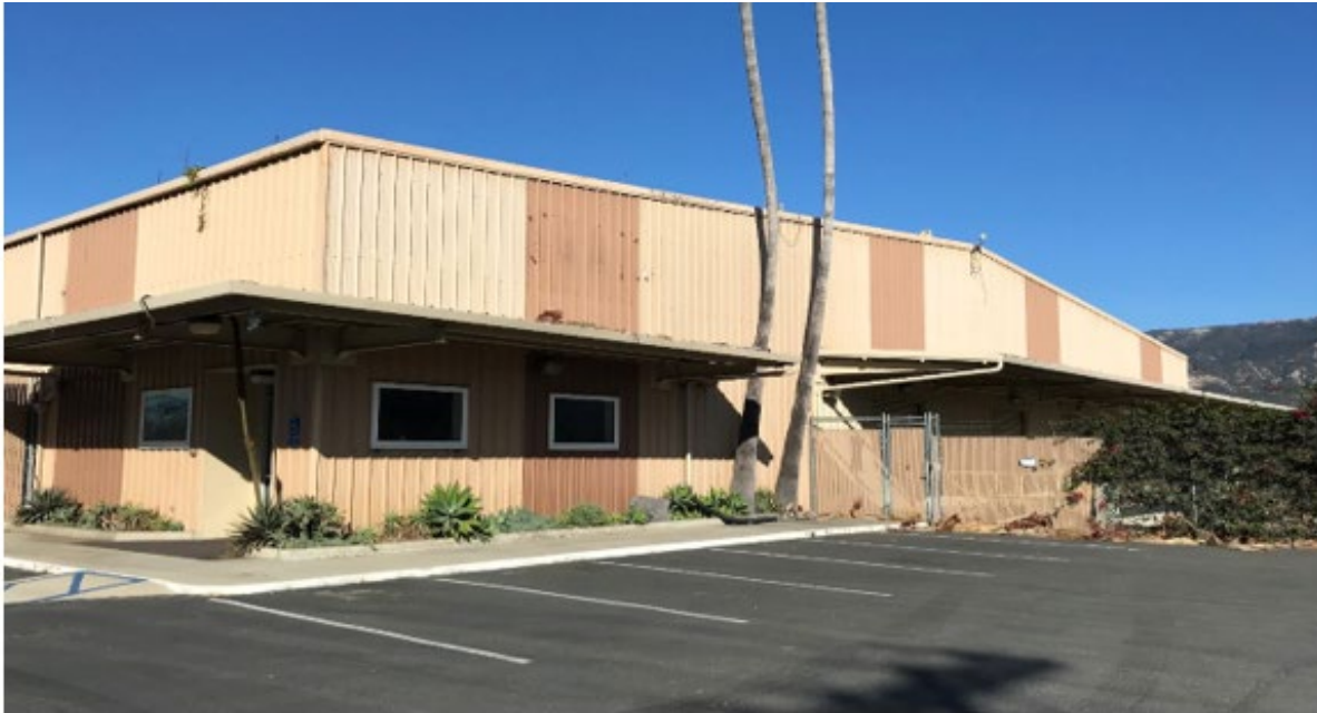
View of the east side of the existing building looking northwest
