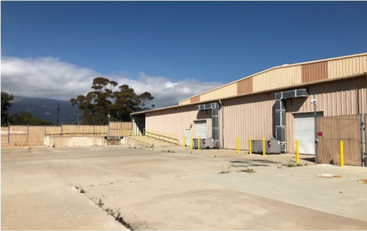
View of the west side of the existing building looking north
