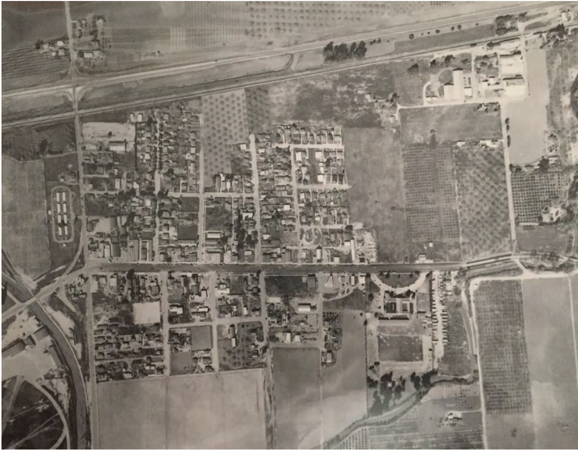
Aerial view of Old Town Goleta, 1952. Source: Goleta Valley Historical Society.
