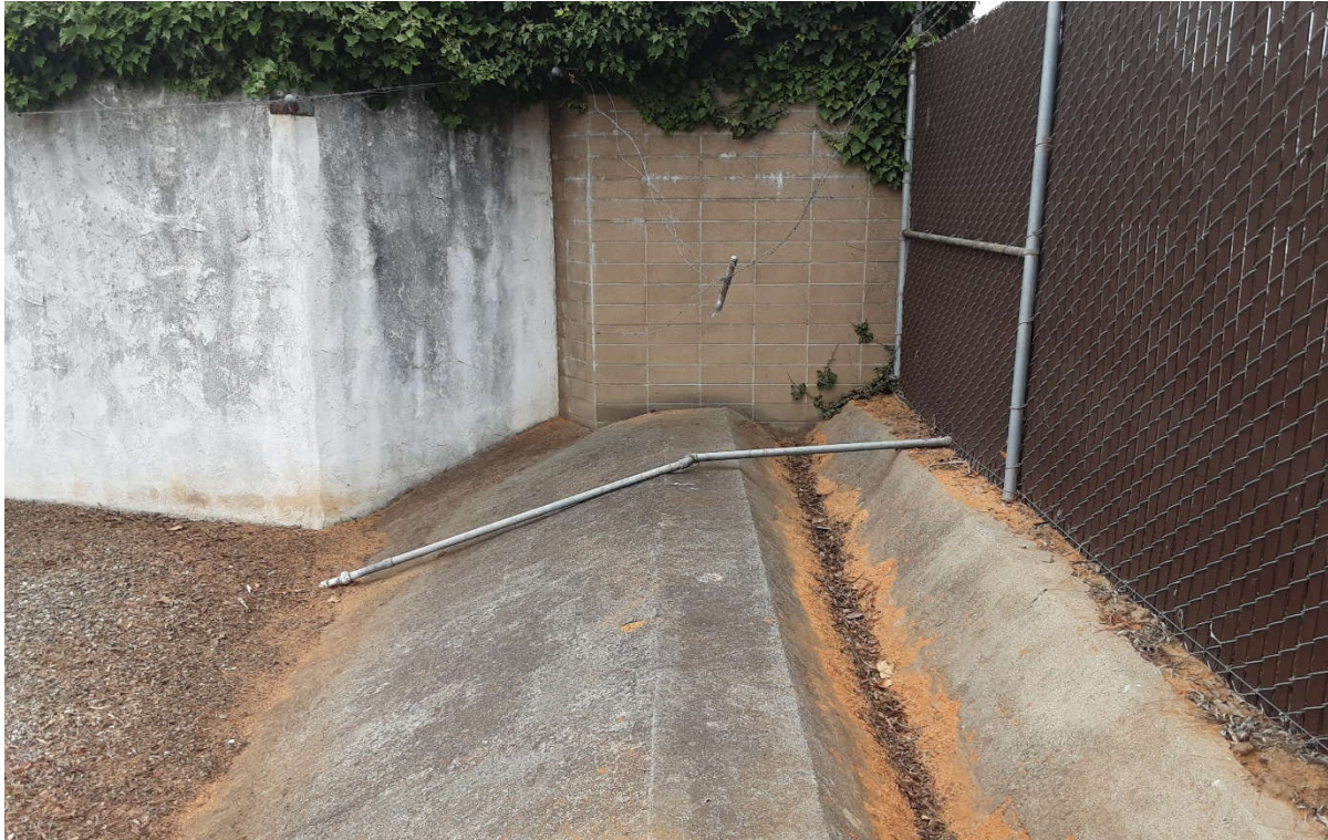
Photograph 7. View of channel in substation at northwest corner.
