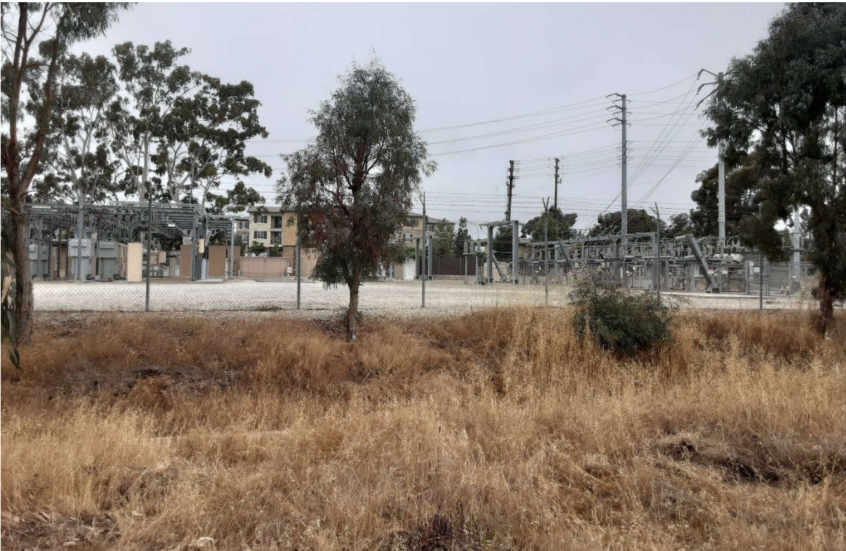
Photograph 2. View of substation and improvement area for hammerhead turnaround, access road, ramp, and swing gate facing west.
