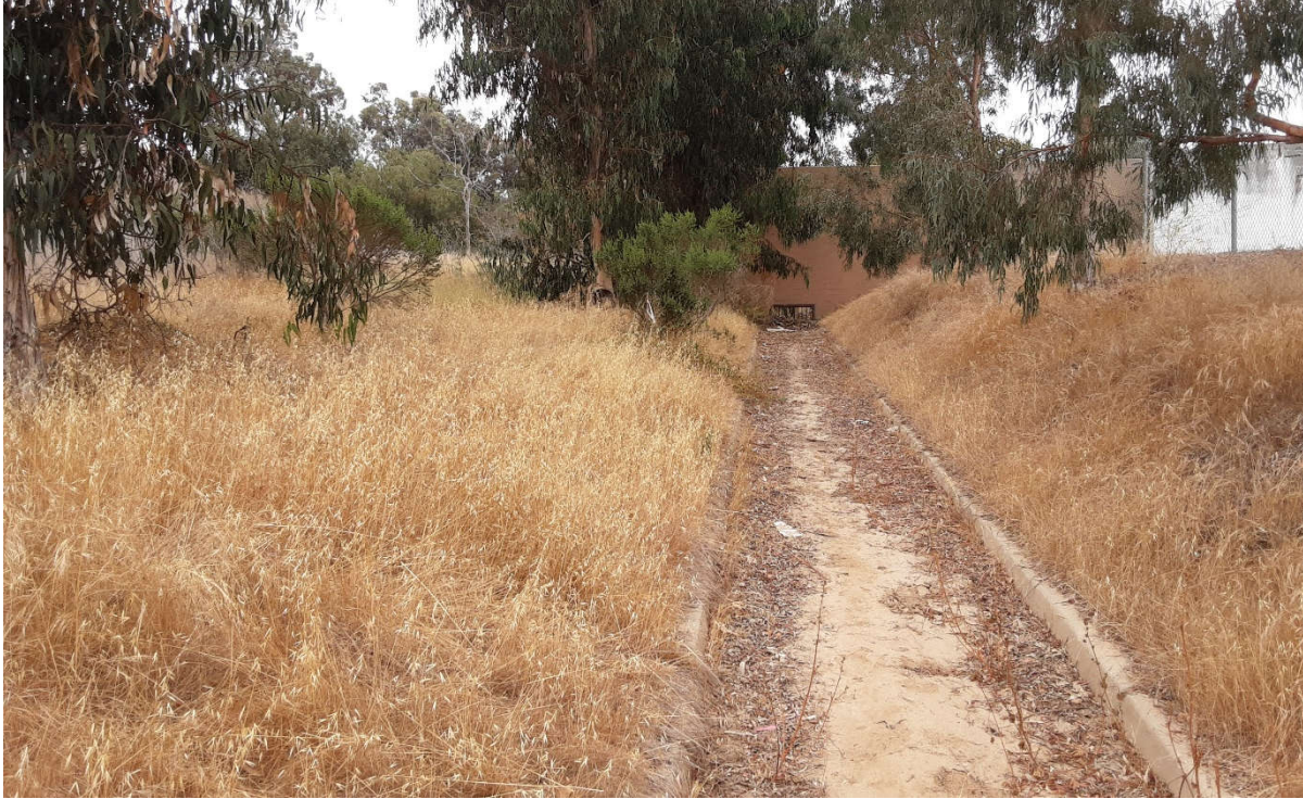
Photograph 3. View of concrete channel facing south.
