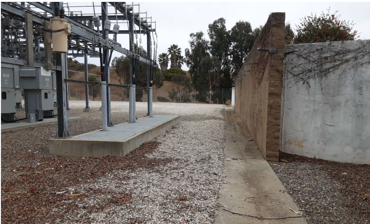
Photograph 8. View of channel within substation along southern side, facing east.
