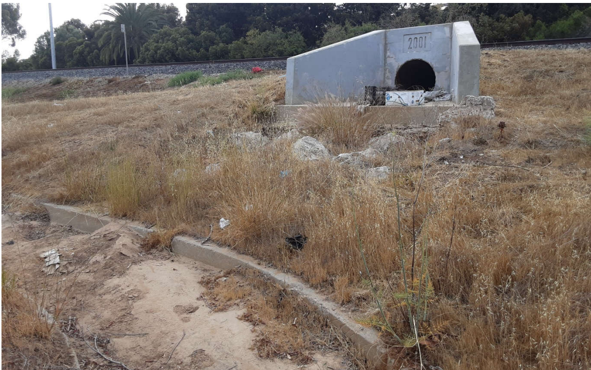
Photograph 4. View of culvert upslope of concrete channel facing north.
