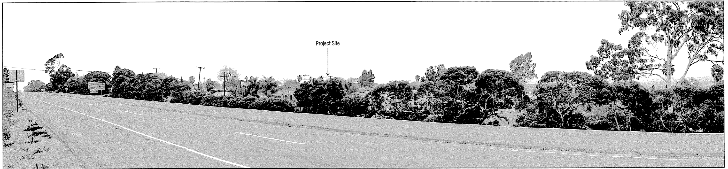
View A – The view shown, although taken from the south side of the 101 Freeway from a location 375 feet southeast of the project site, clearly illustrates the view screening and blocking effects of the landscaping planted within the Caltrans ROW along the north side of the freeway. In views from the westbound lanes the roadside landscaping would coalesce to form a denser visual screen to northerly views. The project site would scarcely be visible from speeding vehicles. In this location views of the mountains would also be effectively screened and blocked by the Caltrans landscaping.
