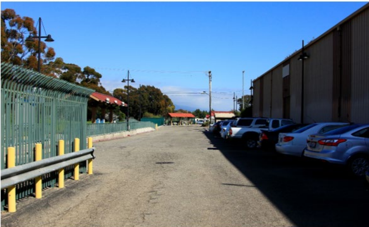
View of the north side of the existing building looking east along the railroad right-of-way
