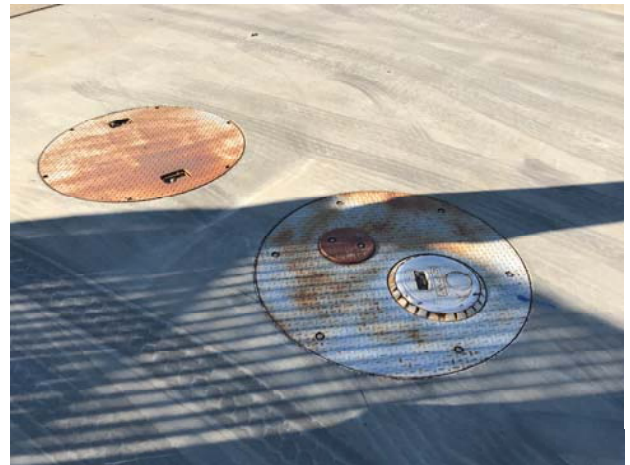
Photograph 6. View of the location of an 1,800-gallon UST in the western portion of the subject property.
