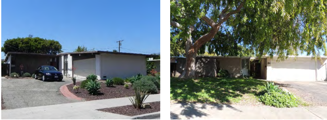
Examples of Kellogg Park homes. Left: 87 Mallard Avenue, August 2016; Right: 84 Mallard Avenue, February 2016. Source for both: Historic Resources Group.
