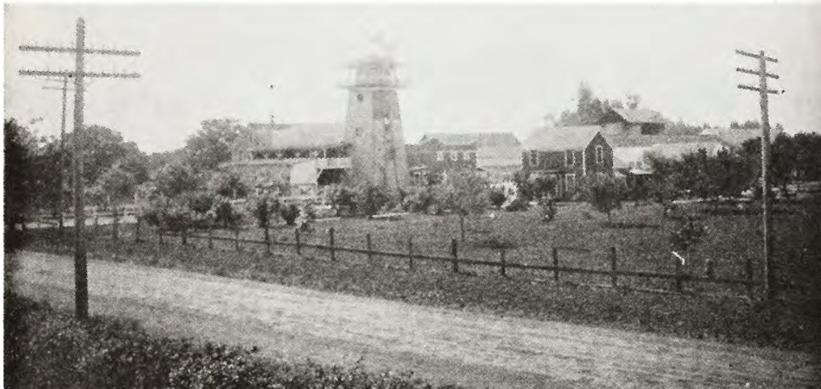
Kellogg Dairy, c. 1900 (demolished). Source: Tompkins, Goleta: The Good Land .
