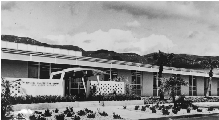
Rendering of Raytheon building (75 Coromar Drive, 1957; Howell, Arendt, Mosher and Grant), 1958. The building does not appear to have been constructed to plan. Source: Local History Collection, Department of Special Collections, University of California at Santa Barbara, Santa Barbara, CA.
