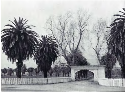
Former entrance to Glen Annie Ranch, including Hollister Arch, n.d. Source: goletahistory.com.
