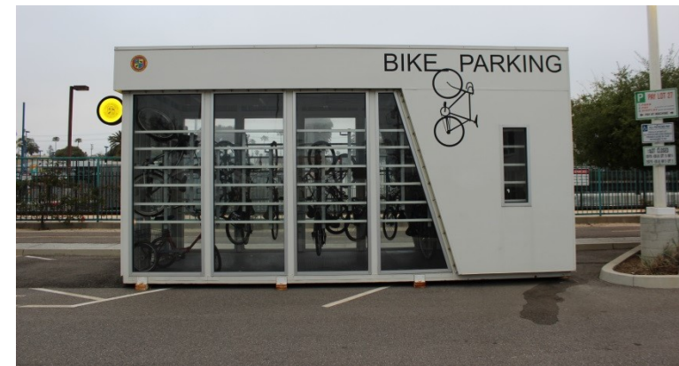
Enclosed bicycle parking, Oceanside, California
