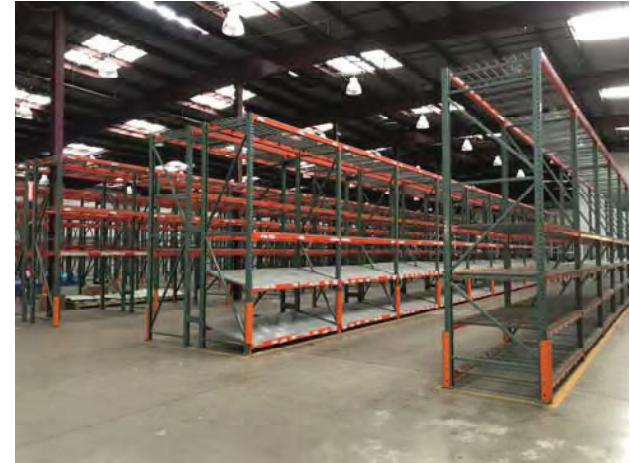
Photograph 3. View of the interior vacant warehouse space on the subject property.
