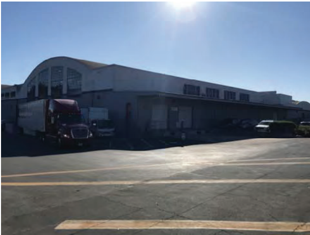
Photograph 10. View of the eastern adjacent multi-business commercial building (30 S. La Patera Lane), facing southeast.
