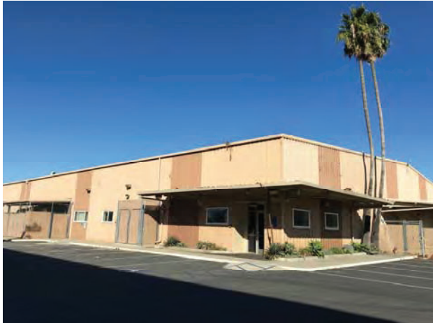
Photograph 1. View of the building on the subject property, facing northwest.
