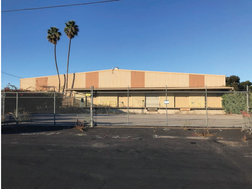
Photograph 1. View of the existing warehouse building in the project site. Photograph taken from the east side of the project site, facing west.
