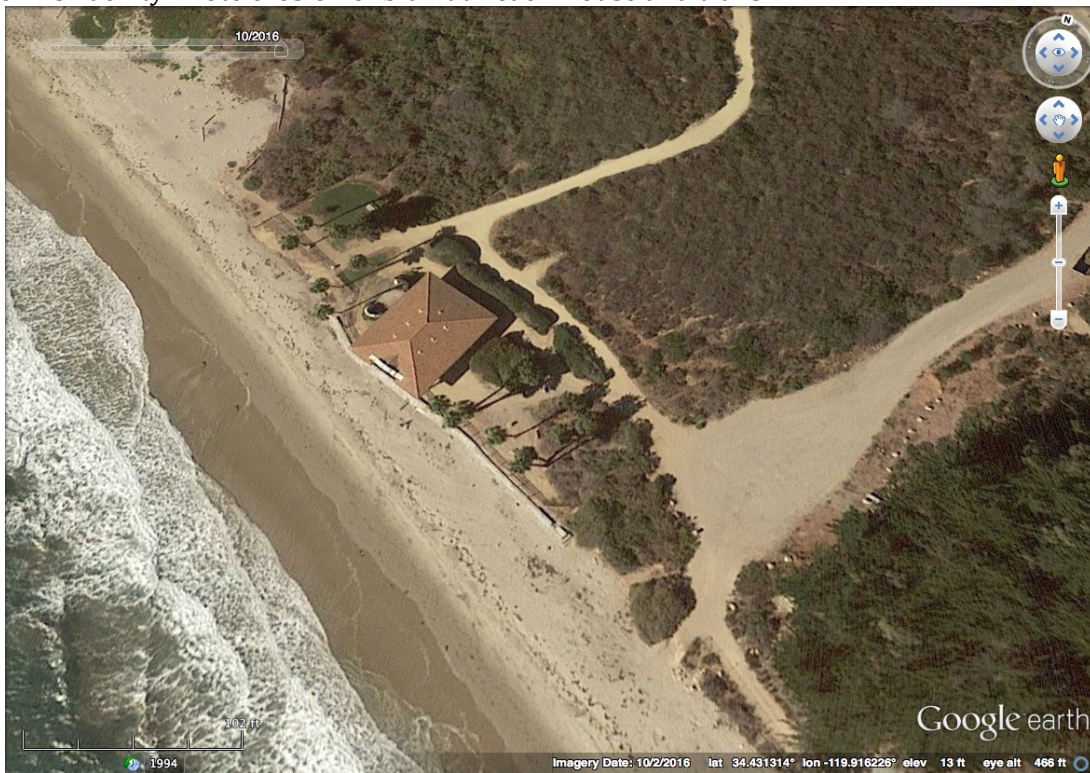
Photo 6. Close up view of Beach House with temporary wall protecting tidal surge and bluff erosion. Note the ruderal/disturbed area along the road edges.
