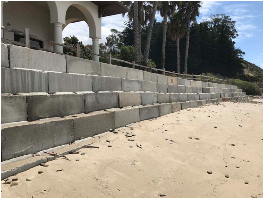
Photo 8. Close up view of the temporary wall protecting the Beach House. Note sand with no exposed cobble in this location.
