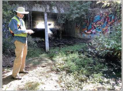
Bridge culvert connecting to downstream concrete channel
