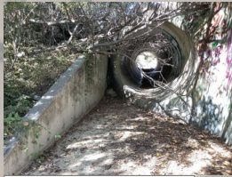
Culvert from Tecolobito into Glen Annie
