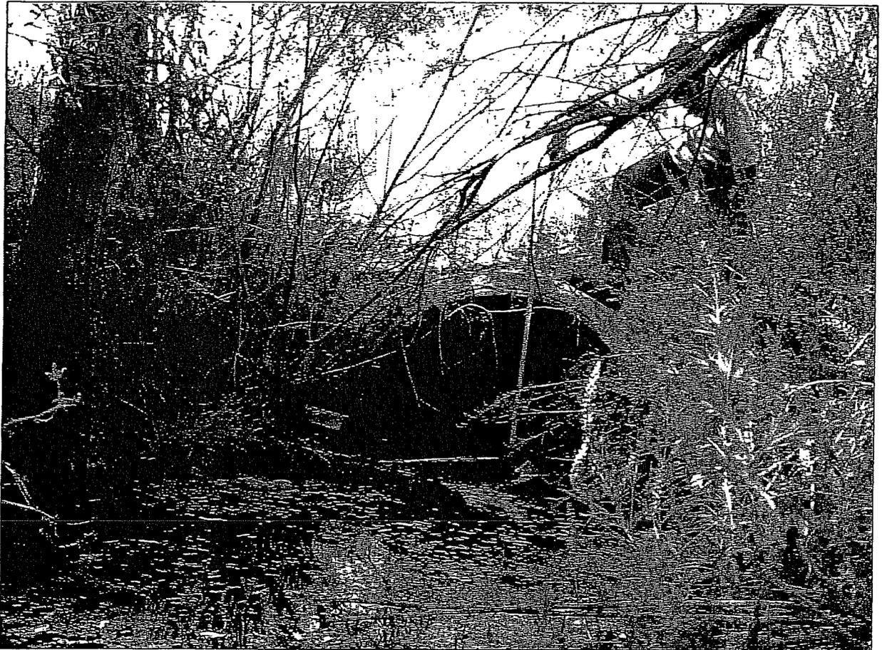
Figure 3-Whittier Drive Storm Drain Discharge Point. The author is using a tape measure to collect measurements of the usable space in the pipe. The discharge pipe is a circular reinforced concrete pipe with a diameter horizontally of 5-feet. The pipe has significant sediment below the water line because the depth to sediment from the top of the pipe is only 3 feet.
