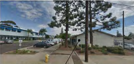
EXISTING BUILDINGS 'B' & 'C' BEYOND TO BE REMOVED
