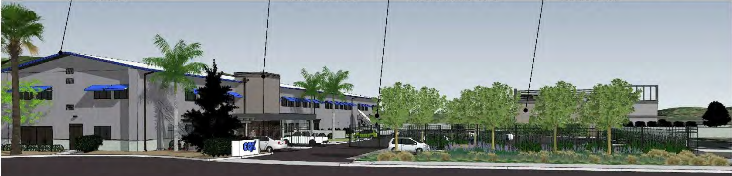
EXISTING ADMIN/OFFICE BUILDING 'C'
