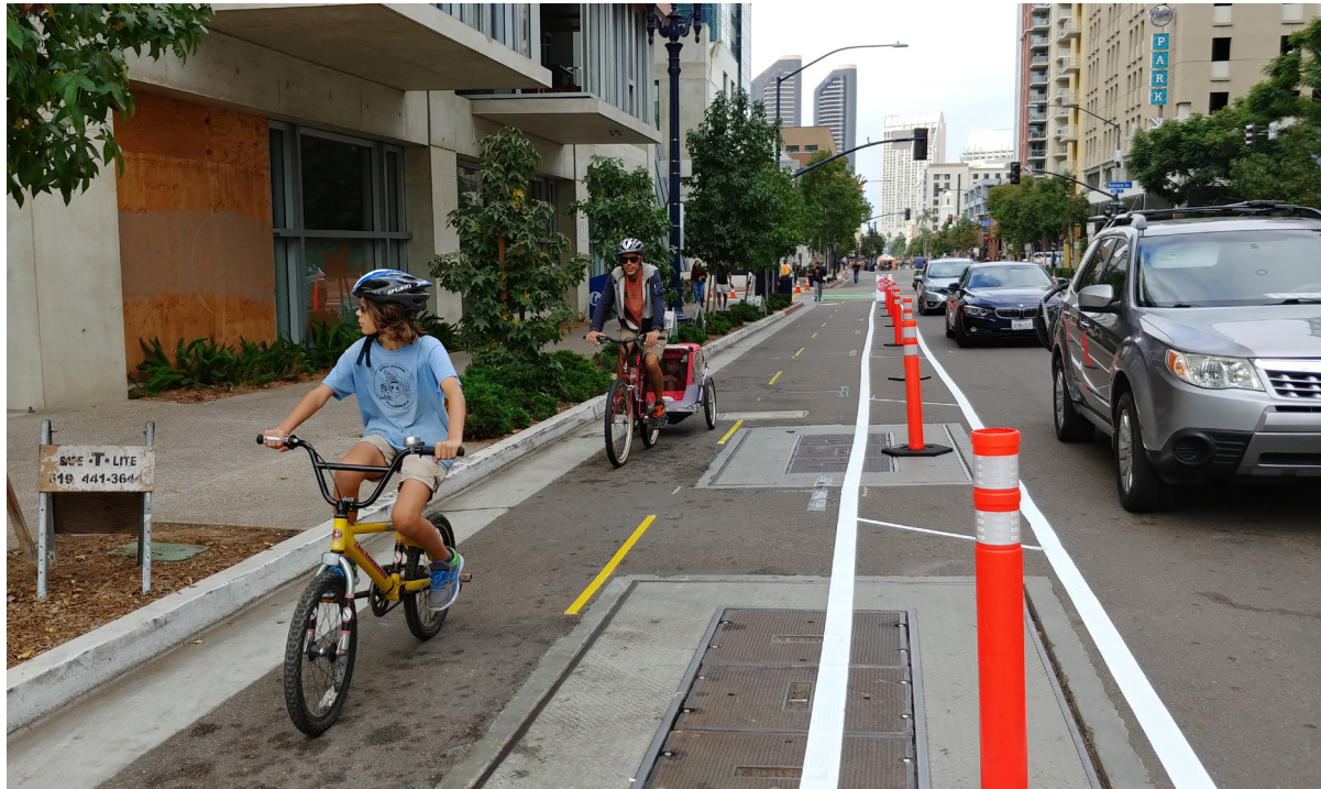
Temporary Cycle Track installation
