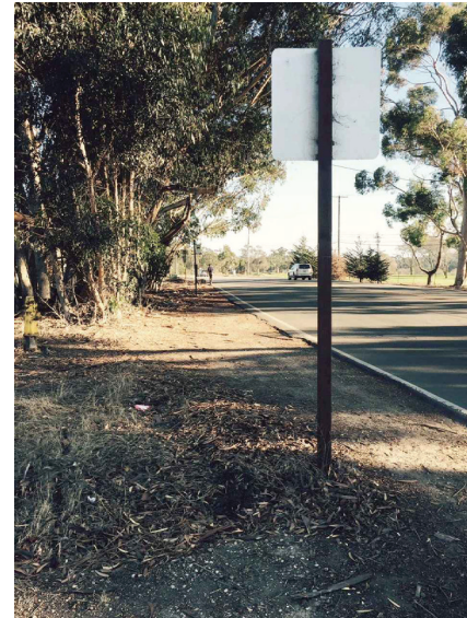
SIGHT DISTANCE LOOKING EAST
