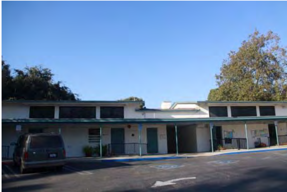
Figure 6 – Building B, Original building to the left, new addition to the right
