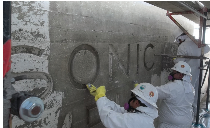
Figure 19. Cleaning and restoring lettering in concrete. Source: Spectra Company.
