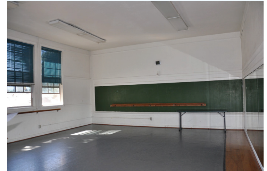
Figure 22. Typical Main Building classroom interior. Finishes can be upgraded and new systems installed without significantly altering the space.
