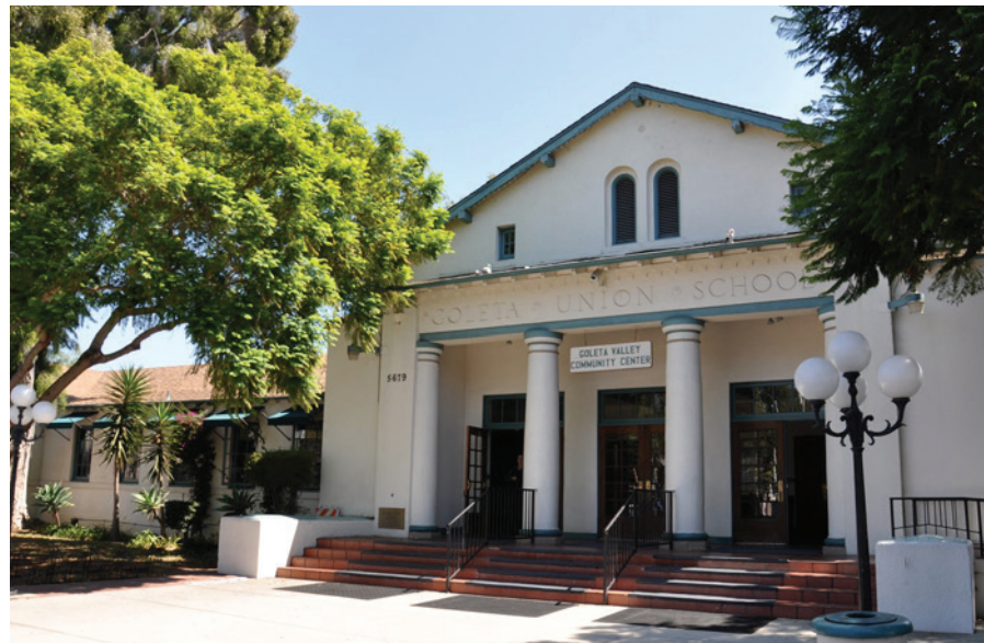
Figure 1. Main Building north facade at main entrance, looking south.
