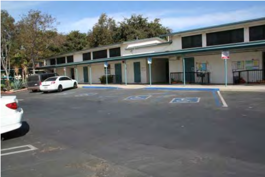
Figure 2 – Front of Building B
