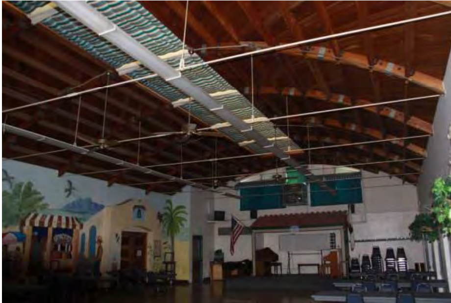
Figure 4 – Building A, Barrel Vaulted Roof Addition
