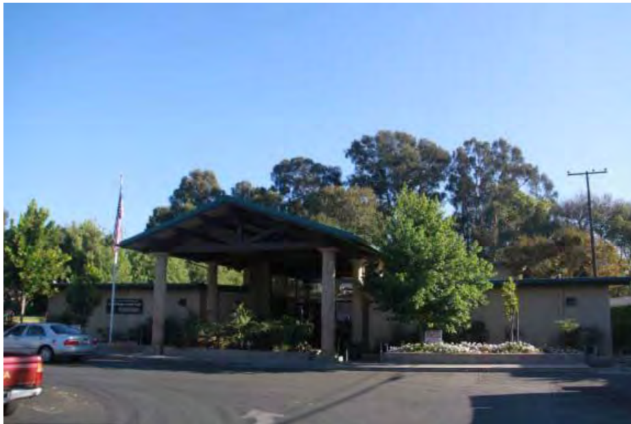
Figure 5 – Front of Building D
