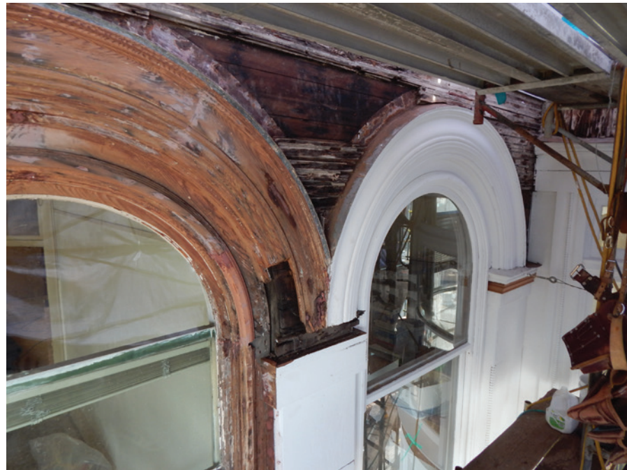
Figure 20. Wood repair and maintenance.
