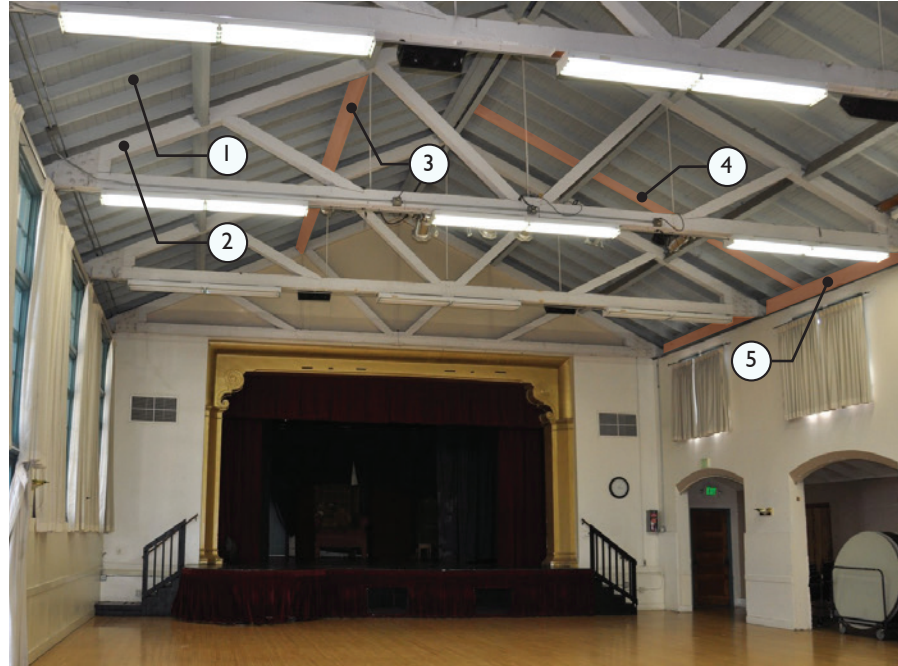
Figure 15. Auditorium, annotated with key framing elements.
