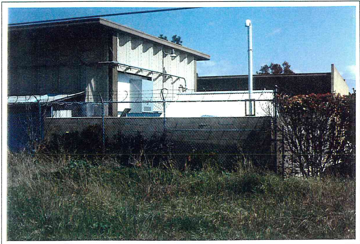
Photo 6. Enclosure and vent pipe on east adjacent property.
