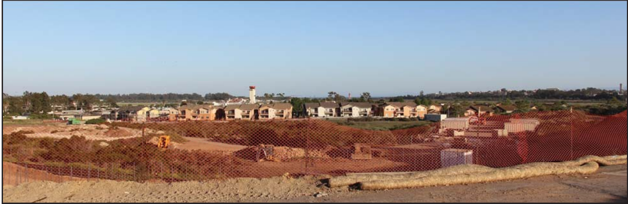
Current Conditions Without Simulated Road Construction
