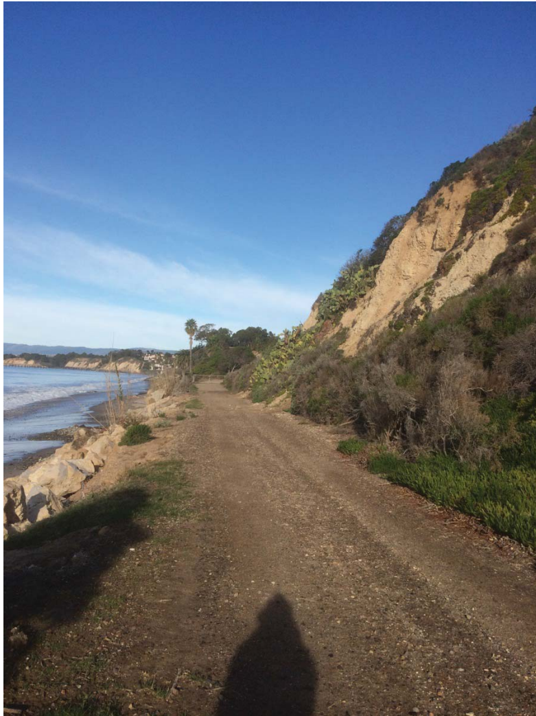
Photo 1. Western portion of access road, looking west toward road entrance gate.
