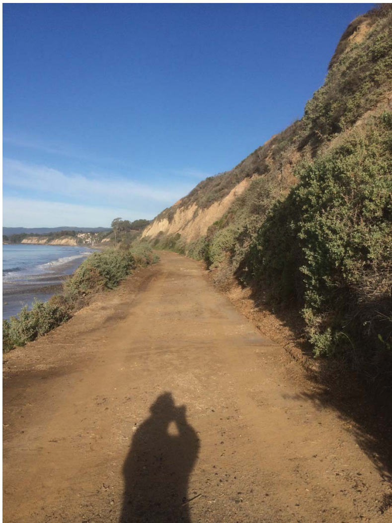
Photo 3. Central portion of access road, looking west, near entrance to PRC 421-1.
