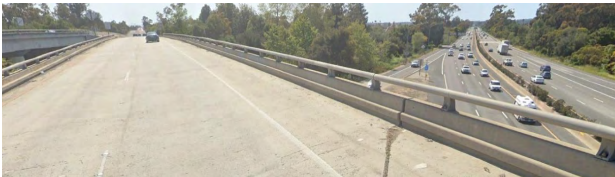
Figure A-10. SR 217 over US 101 facing south (Source: Google Earth, 2020)
