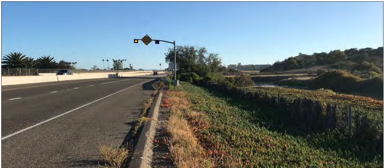
Figure A-7. SR 217 facing southwest
