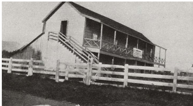
Birabent Hotel, n.d. The Birabent Hotel (1870; demolished) was for many years the largest building in La Patera. Source: Tompkins, Goleta: The Good Land .
