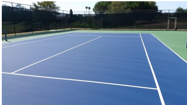
Evergreen Tennis Court Resurfaced
